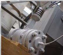
Thermal fins to isolate the stem tightness from the cold temperature
